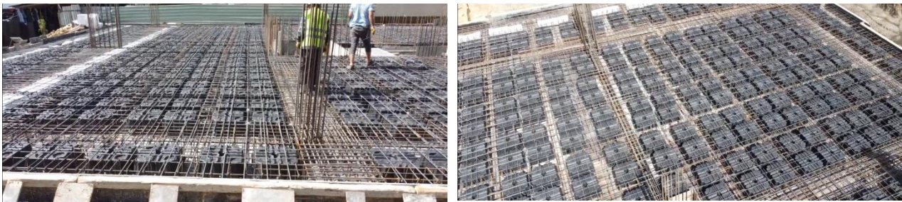
Figure 1. Placement of prismatic cavities forming cavities
